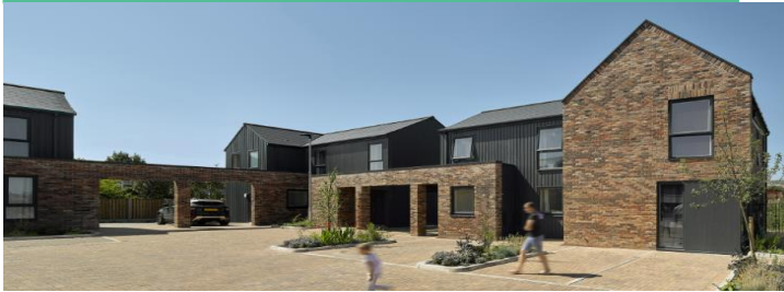
Each house type is bespoke around a communal courtyard, encouraging interaction between residents
